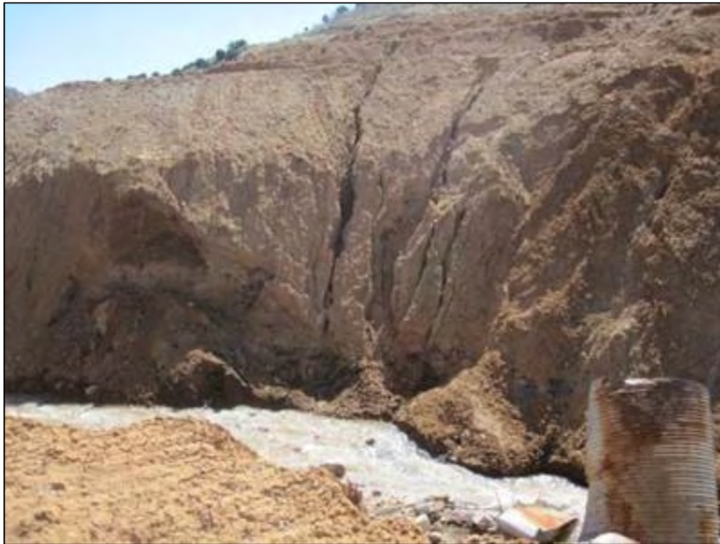
Figure 27. Streambank erosion occurring in the South Fork Chalk Creek subwatershed.
